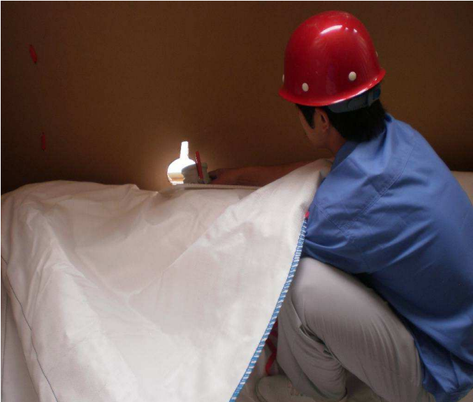
12. Put the valve through the valve hole
